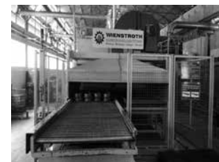
Fig 2.9 View of Wienstroth Furnace
